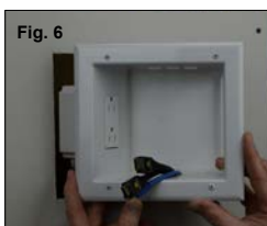
Figure 6: Important: Before installing the Expandable Media Plate into the template opening, make sure to pull your low voltage cables through the low voltage cable opening.
