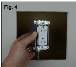
Figure 4: Connect the supplied 20 Amp Duplex Receptacle to a piece of 14/2 with ground UL approved electrical building wire that you have pulled from a power source. Strip off approximately 3 inches of the outer jacket of the wire. Be careful not to cut the jacket of the inner wires. Connect the hot line (black) wire to the brass colored terminal screw and neutral (white) wire to the silver colored terminal screw. Be sure to connect the grounding (green) or bare grounding wire to the green colored terminal screw. Once you have wired the 20 Amp Duplex Receptacle, screw it into the Steel Electrical Box until the receptacle is firmly secured.
