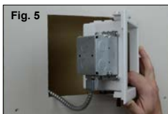
Figure 5: Use the four provided screws to secure the Steel Electrical Box and Receptacle to the mounting studs on the backside of the Expandable Media Box.
